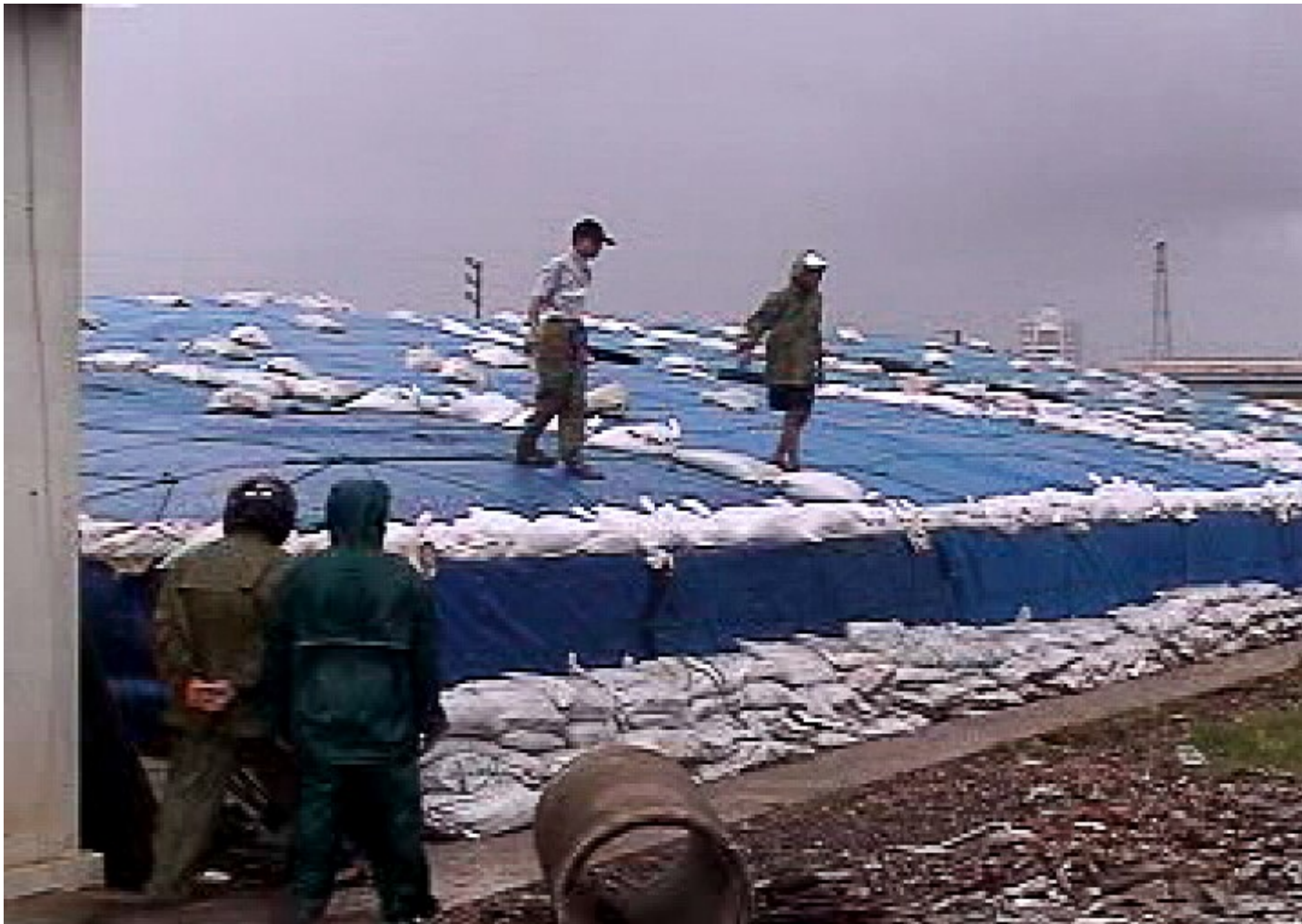
Pic 05: Anti-storm activities at the salt plant
