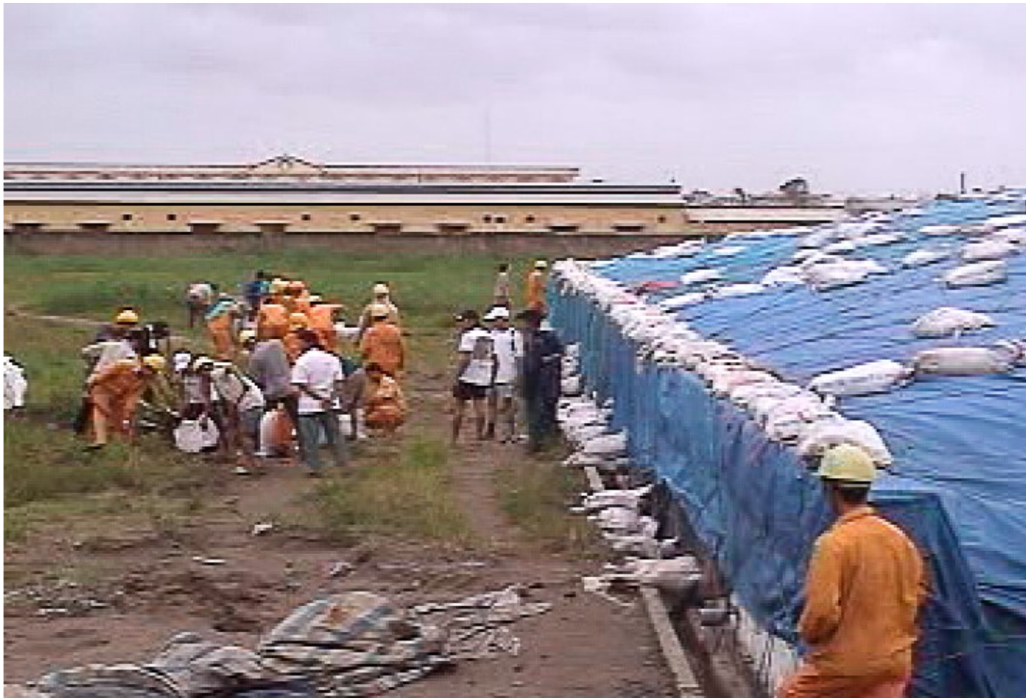
Pic 03: Anti-storm activities at the salt plant
