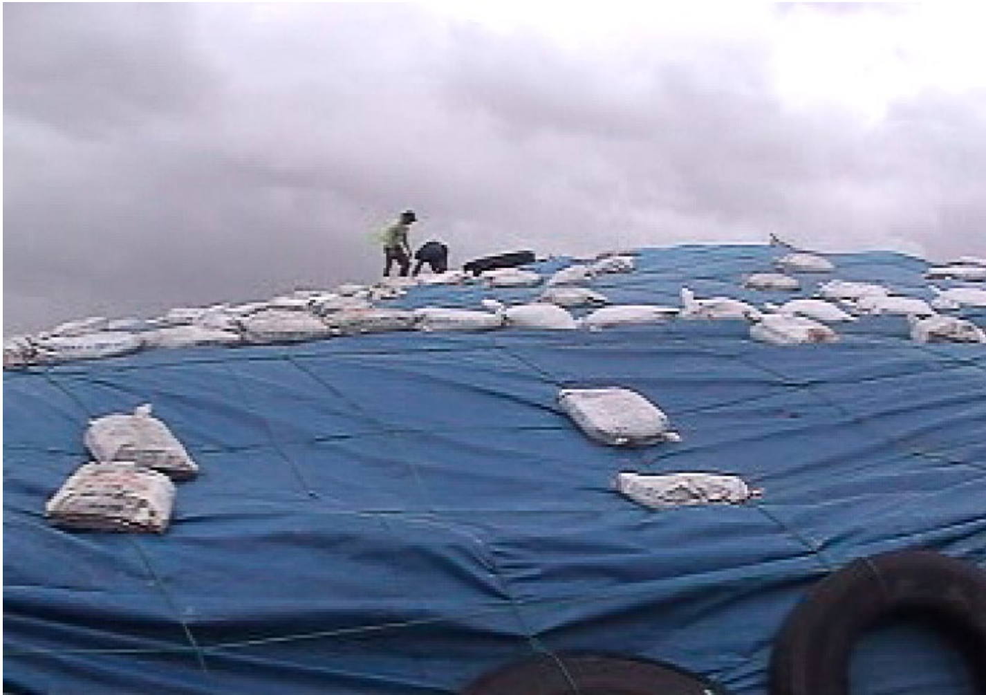
Pic 07: Anti-storm activities at the salt plant
