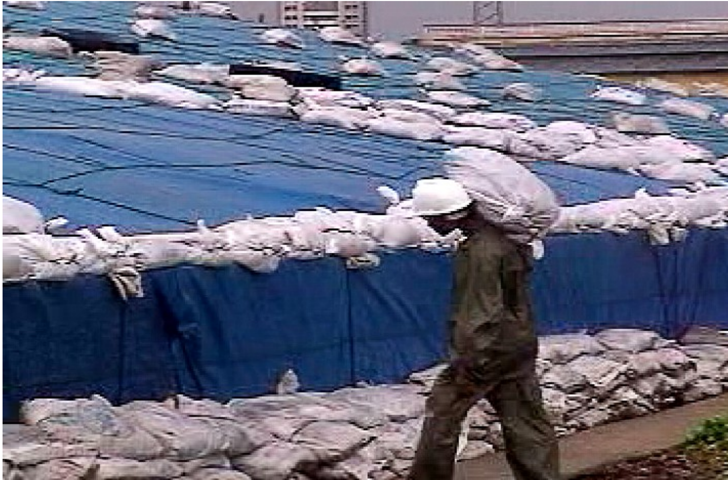
Pic 04: Anti-storm activities at the salt plant
