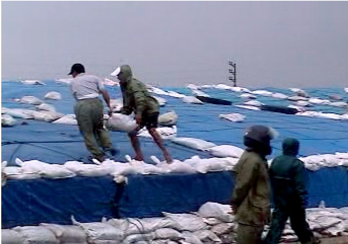
Pic 06: Anti-storm activities at the salt plant
